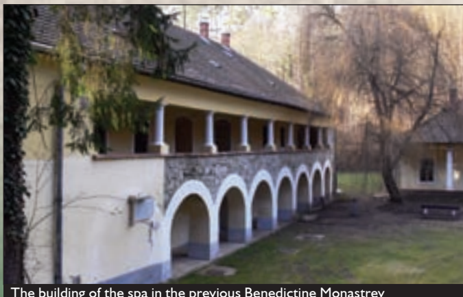
The building of the spa in the previous Benedictine Monastery
